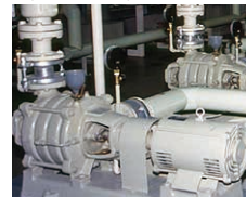
■ Existing water supply pumps (5.5kW × 2)
