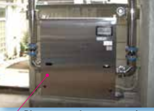
Direct connection water supply booster pump
