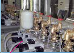
Pressurized water supply pump
